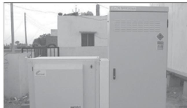
During the recent difficult circumstances presented by Hurricane Sandy, 17 Ballard ElectraGen™-ME systems provided critical electricity to the Bahamas mobile telephone network when the storm downed power lines and cut off grid power. In the three days that Hurricane Sandy passed over the Bahamas, each of the 5kW systems operated flawlessly.
