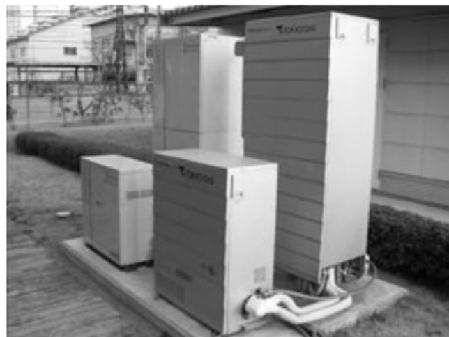
Superior Products Award for Excellence 2012. The annual award recognizes new products and services. Eneos' solid oxide fuel cell was introduced into the Japanese Ene-Farm residential fuel cell scheme in October 2011 and cogenerates electricity and heat using city gas. The 700W systems boast a power generation efficiency of 45% and can provide up to 70% of the power requirement for the average home. It is currently sold for ¥2.7 million (\$31,000) and comes with a 10 year warranty.
