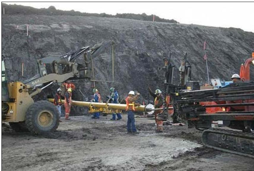
A crew installs a casing into oil sands at a test site in this photo. The casing surrounds an antenna that is inserted into the sand
